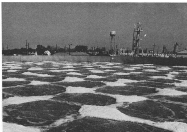
Figure 1. Typical waste water treatment facility. (Photograph courtesy of Virginia Chemicals.)
